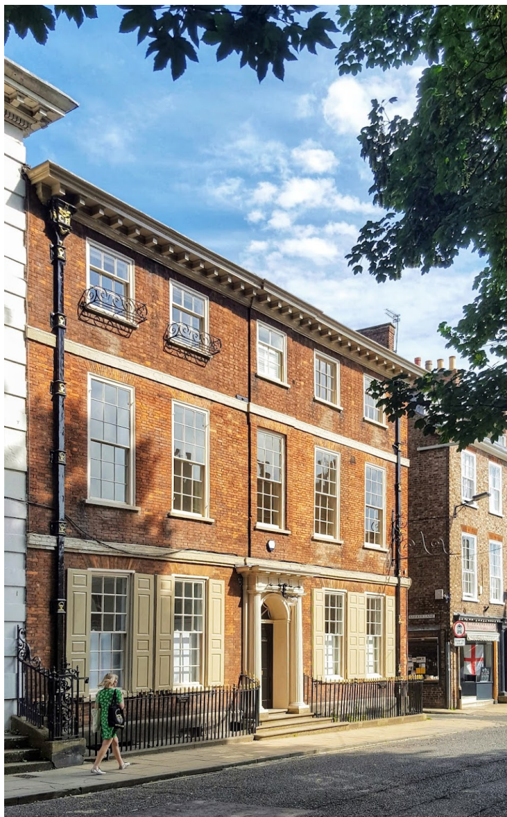
This house in York would probably be inconsistent with Part O rules on overheating (clauses 1.7 and 1.10) and certainly on window guarding (clause 3.9). But should the Government really stop British people from building houses like this if they want to?
